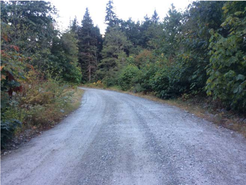
Left approach viewed from bridge
